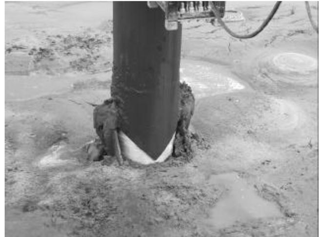
Figure 5. Installed column after drawing the steel pipe under vibration
