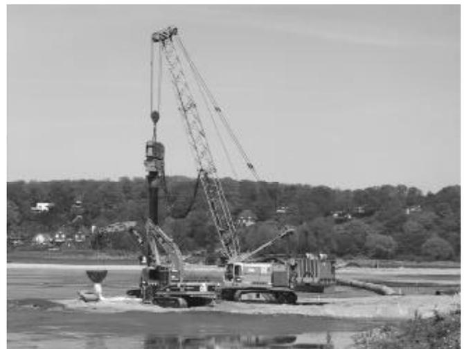
Figure 6. The well-tested vibro displacement method on land.
