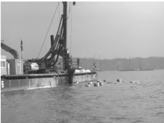
Figure 4. Installation by vibro displacement from offshore pontoon
