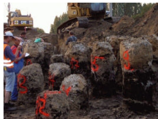
Fig. 6. Excavated columns with different heights
