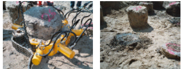
Fig. 11. Cutting the pile heads
