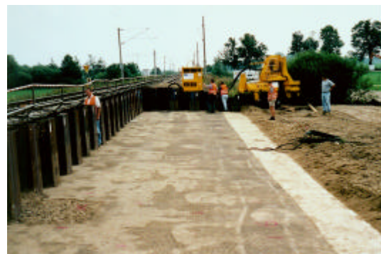
Fig. 5. Temporary sheet pile walls and excavated embankment in the test field
