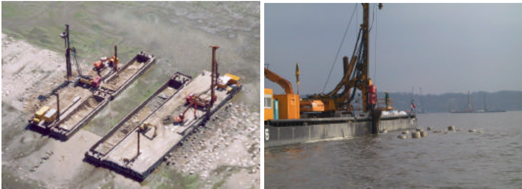
Figure 3. Column installation in hydraulic engineering
