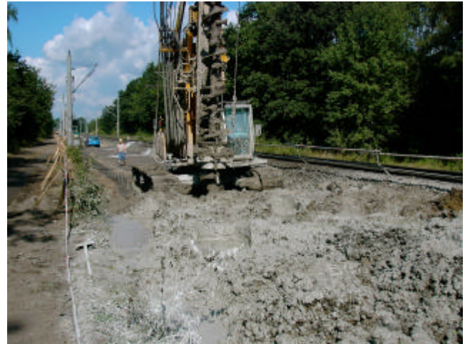
Figure 6. Installation of MIP-columns.
