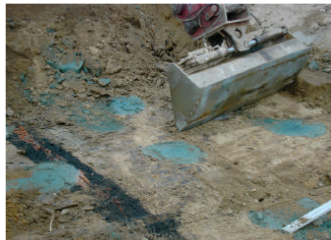
Figure 7. Shortening of the MIP-columns.
