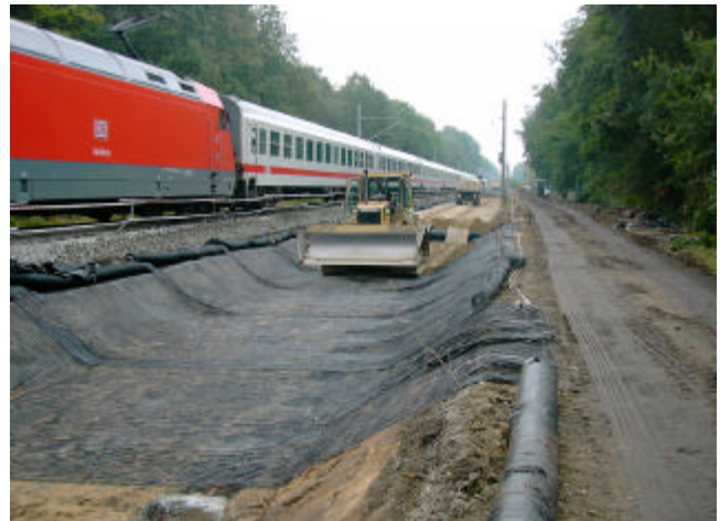
Figure 12. Placing of geogrids.
