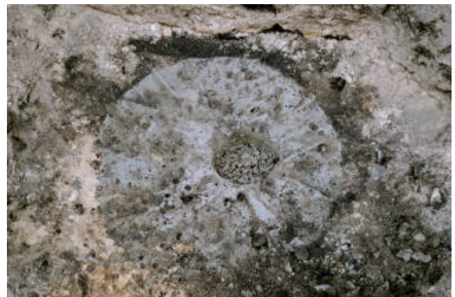
Figure 10. Column after liner extension.
