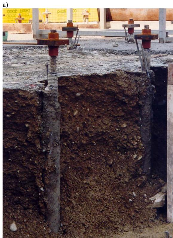
Figure 5. Exposed micropiles with plates at head
