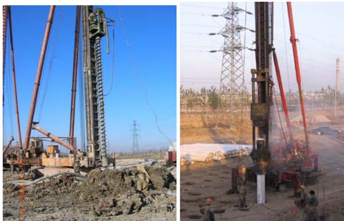
Figure 2. Continuous flight augers and centrifugally precast concrete driven piles.
