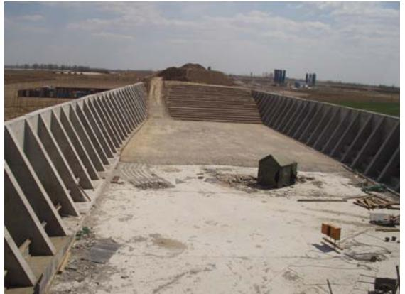
Figure 4. Construction of retaining walls.
