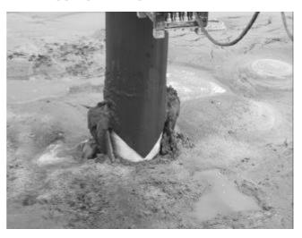
Figure 5. Installed column after drawing the steel pipe under vibration
