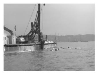
Figure 4. Installation by vibro displacement from offshore pontoon
