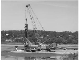
Figure 6. The well-tested vibro displacement method on land.
