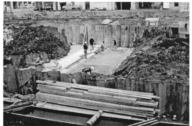
Fig. 5. Excavation and placement of the bottom slab in slices.
