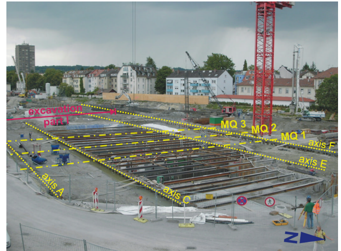
Fig. 8. Execution of the middle strip till block 2 (Axes C-E)
