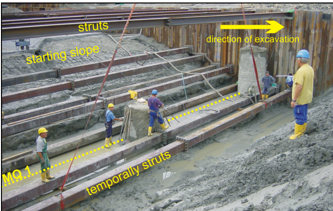
Fig. 11. Details of construction work (axis C-E)
