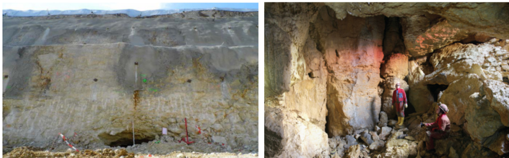
Fig. 8. Cave in a slope of the building pit at the Widderstall tunnel
